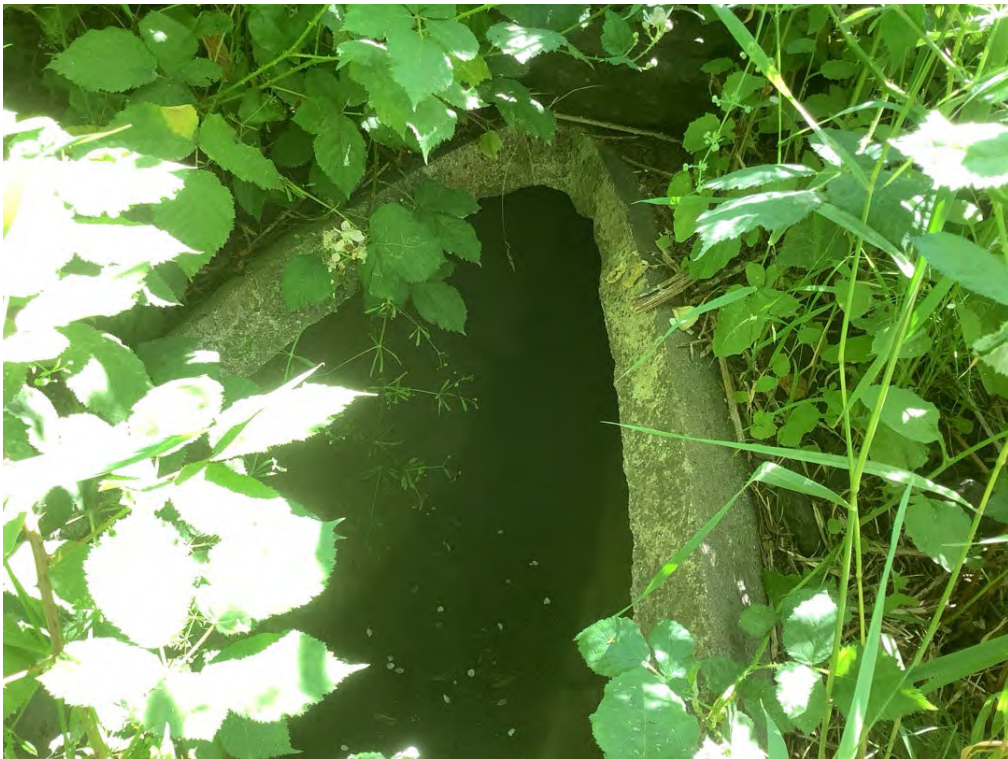
Photo 10. Outlet of on-site stream at culvert under Mullis Street
