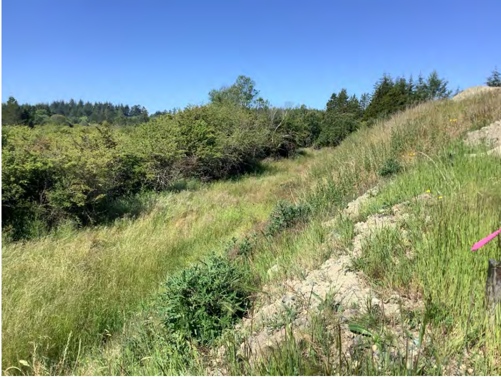
Photo 5. Excavated material and typical vegetation in location of proposed hangars
