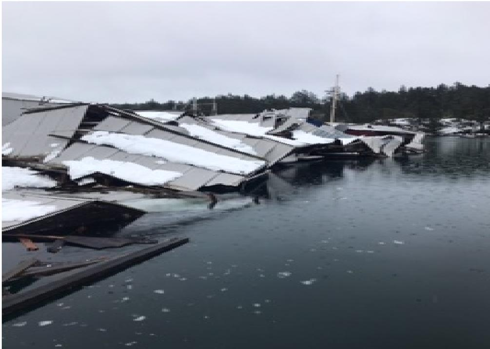
Jensen's Marina took a big hit this week with the collapse of a line of boathouses. The collapse was caused by a combination of heavy snow and rain in a winter storm that arrived in the Puget Sound area the evening of February 12, 2021.
