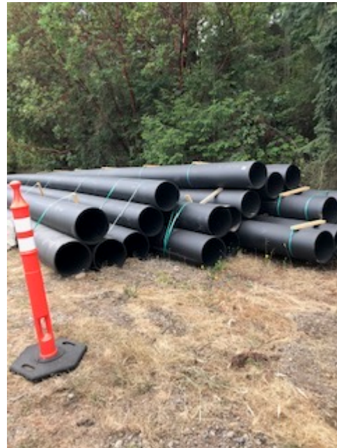
18" HDPE pipe for dock pontoons
