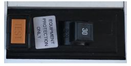
Part of the upgrades to G & H docks are modern shore power pedestals, and with them comes updated electrical code requirements. Similar to the ubiquitous GFCI (Ground Fault Circuit Interrupter) outlet that we're all familiar with finding next to bathroom sinks and on outdoor outlets, the new pedestals are equipped with ELCI (Equipment Leakage Circuit Interrupter) breakers. This means the outlets are now protected by a type of breaker
