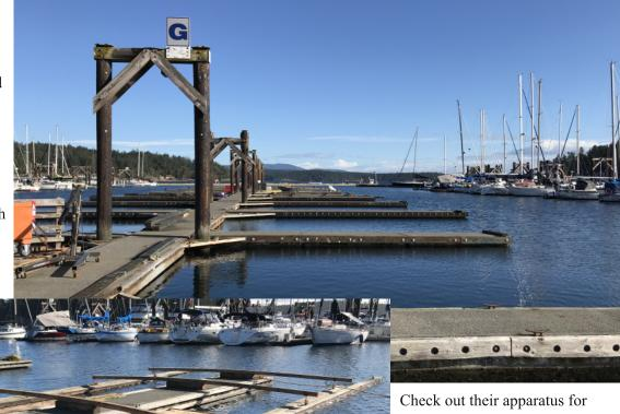
Check out their apparatus for holding those floats in place and upright while they're detached! No you're not seeing things, those are some of the old whalers being used as outriggers. They can then simply float the old boards right out and bring new ones into place.
