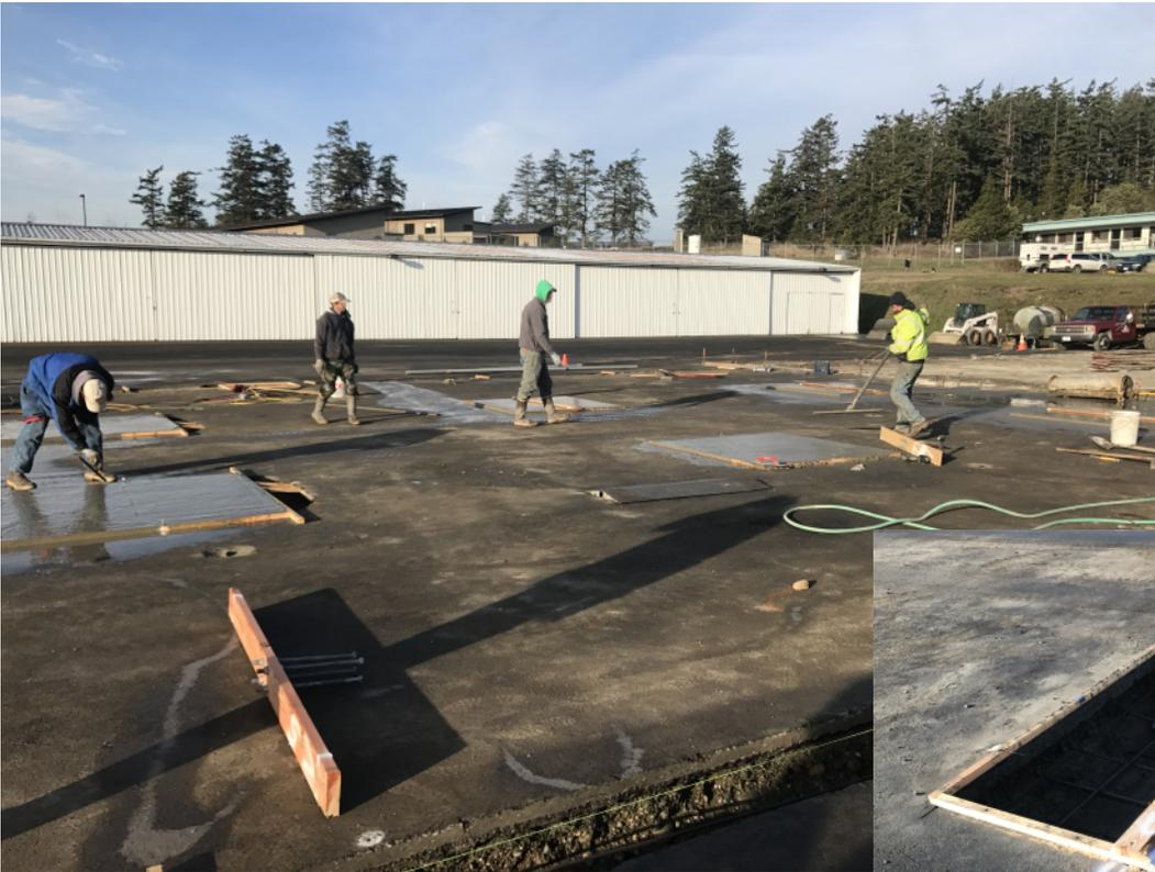
The Maintenance Staff have been hard at work building forms, tying rebar, and dodging weather between concrete pours. The pads for the interior posts are now complete and this week the perimeter footing is being poured. It won't be long now before the structure starts going up! As you can see from the photos, rather than tearing
