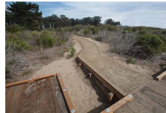
Crushed rock path and wood boardwalk
