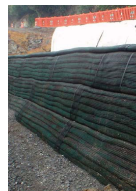
MSE wall prior to rockery installation
