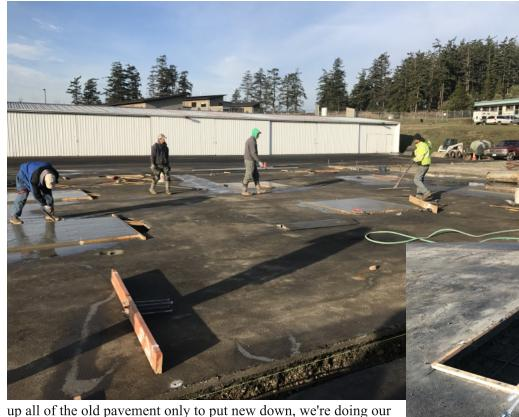
The Maintenance Staff have been hard at work building forms, tying rebar, and dodging weather between concrete pours. The pads for the interior posts are now complete and this week the perimeter footing is being poured. It won't be long now before the structure starts going up! As you can see from the photos, rather than tearing
